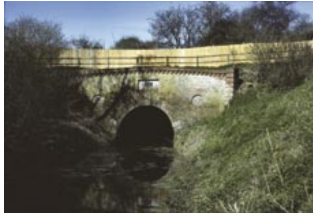
Greywell canal tunnel grille.
