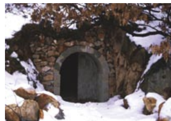
Király-bányák mine entrance after reconstruction and improvement.
