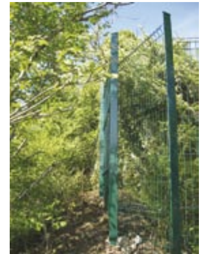
Security fence, France.
