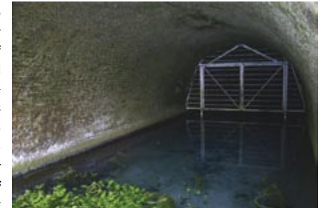
Entrance to Greywell canal tunnel.
